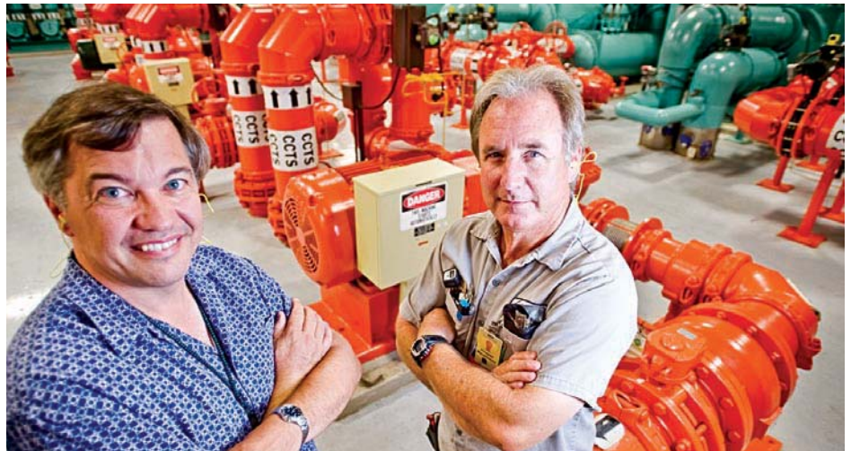
PHOTO: Site Services engineer Art Kienle (left) and mechanic Doug Macpherson helped replicate water and cost savings from Kent, Wash., to El Segundo, Calif. GLADYS WICKERING/BOEING
