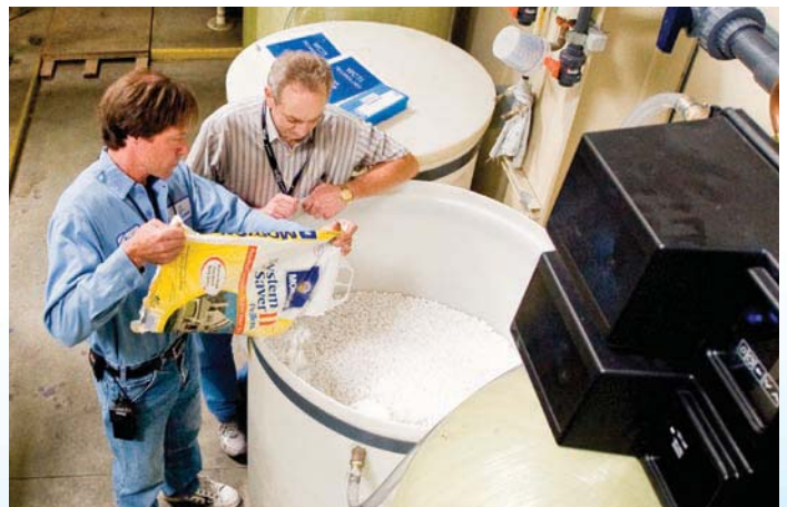
PHOTO: Boeing heating, ventilation and air-conditioning mechanic Brett Weberg adds salt to the regeneration tank for cooling-tower water softeners at the Kent, Wash., site. The water softener is part of a new process initiated by lead mechanical engineer Roger Sampair (right) that will save water and reduce sewage and maintenance costs across Boeing. MARIAN LOCKHART/BOEING
